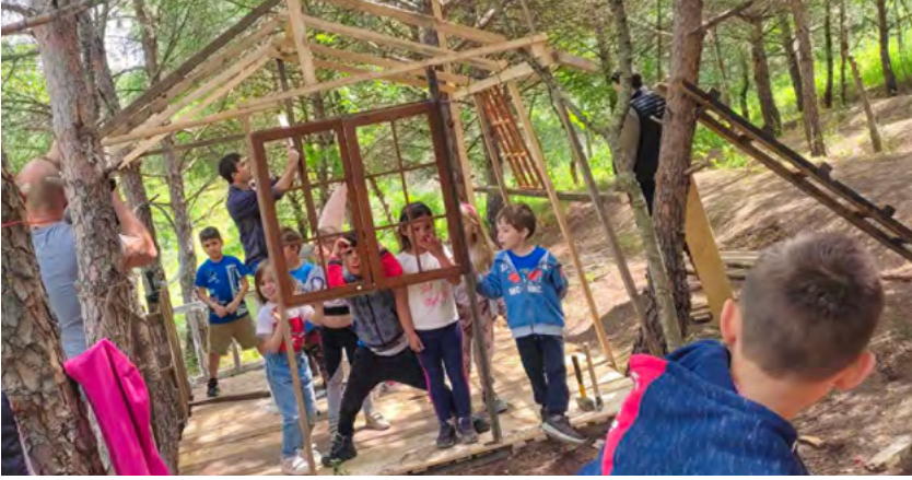
Figure 3.13. Building the “House in the Forest” collectively.
